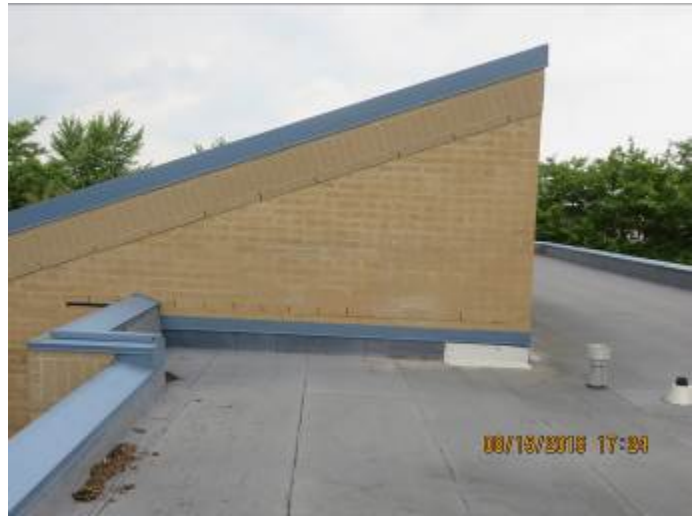
Area 'D' (Thru-Wall Flashing Retrofit)
