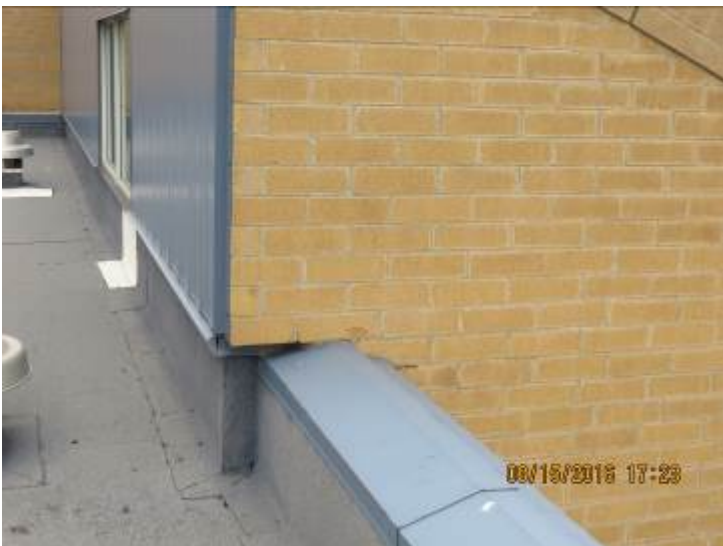
Area 'B' (Thru-Wall Flashing Retrofit)
