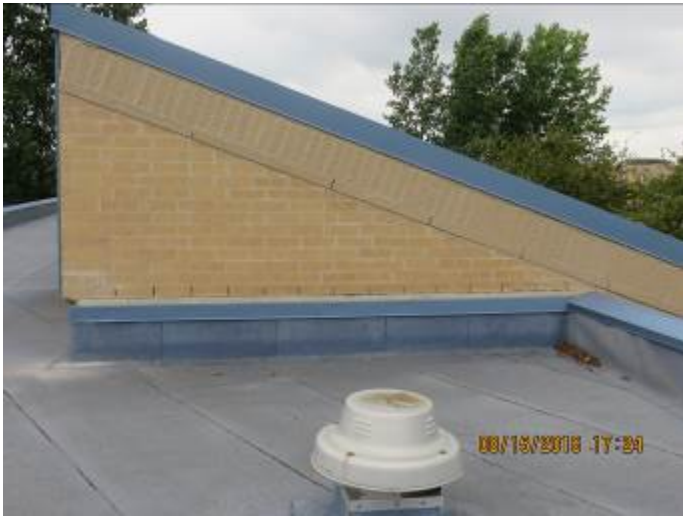
Area 'C' (Thru-Wall Flashing Retrofit)
