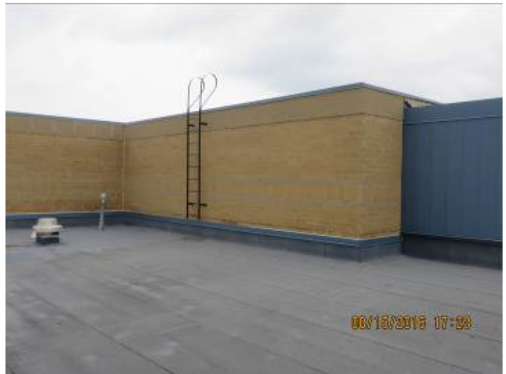
Area 'A' (Thru- Wall Flashing Retrofit)
