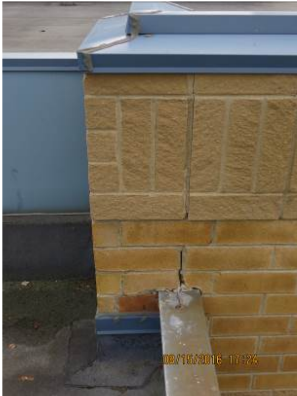
Area 'F' (Soft Joint Construction)
