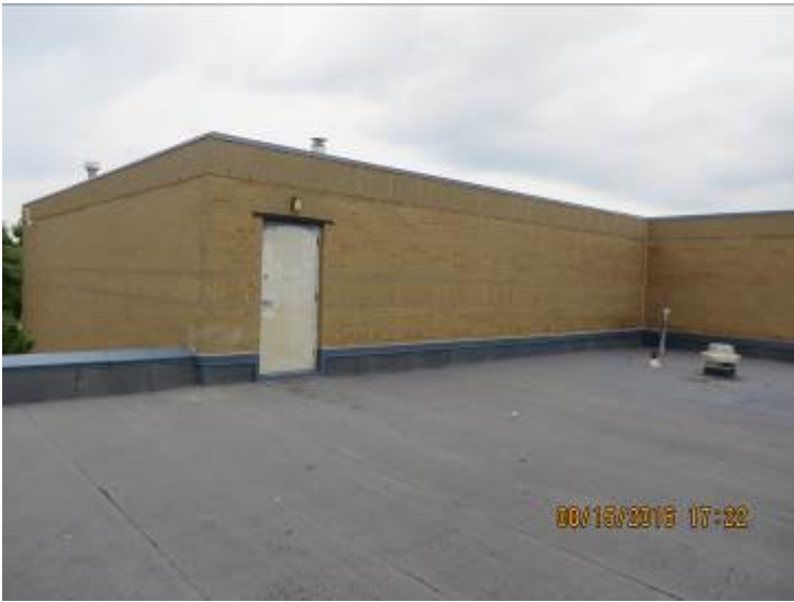
Area 'A' (Thru-Wall Flashing Retrofit)
