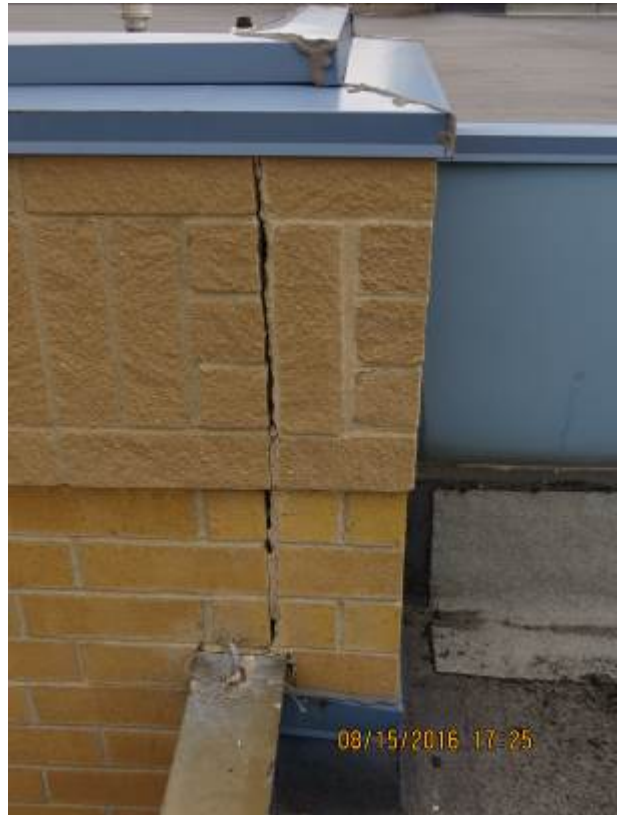
Area 'E' (Soft Joint Construction)
